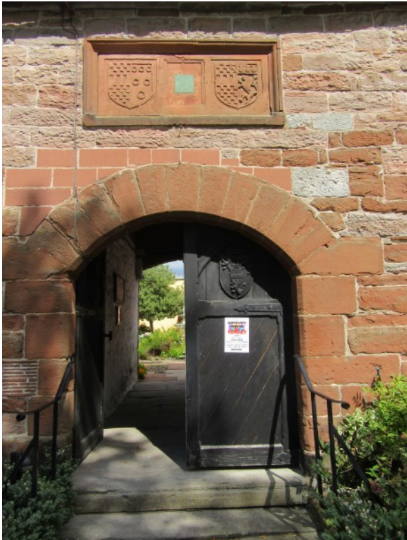
Entrance to the Almshouses at Appleby.
