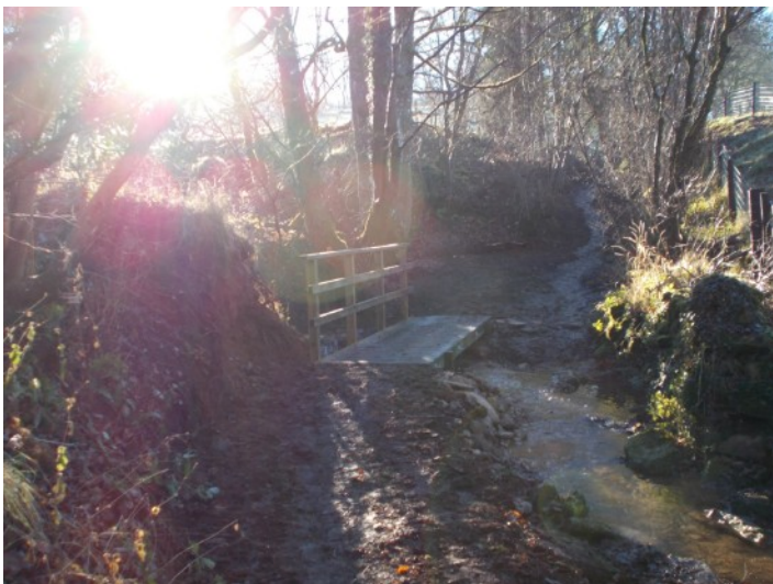
Hartley Lane with new bridge installed.
